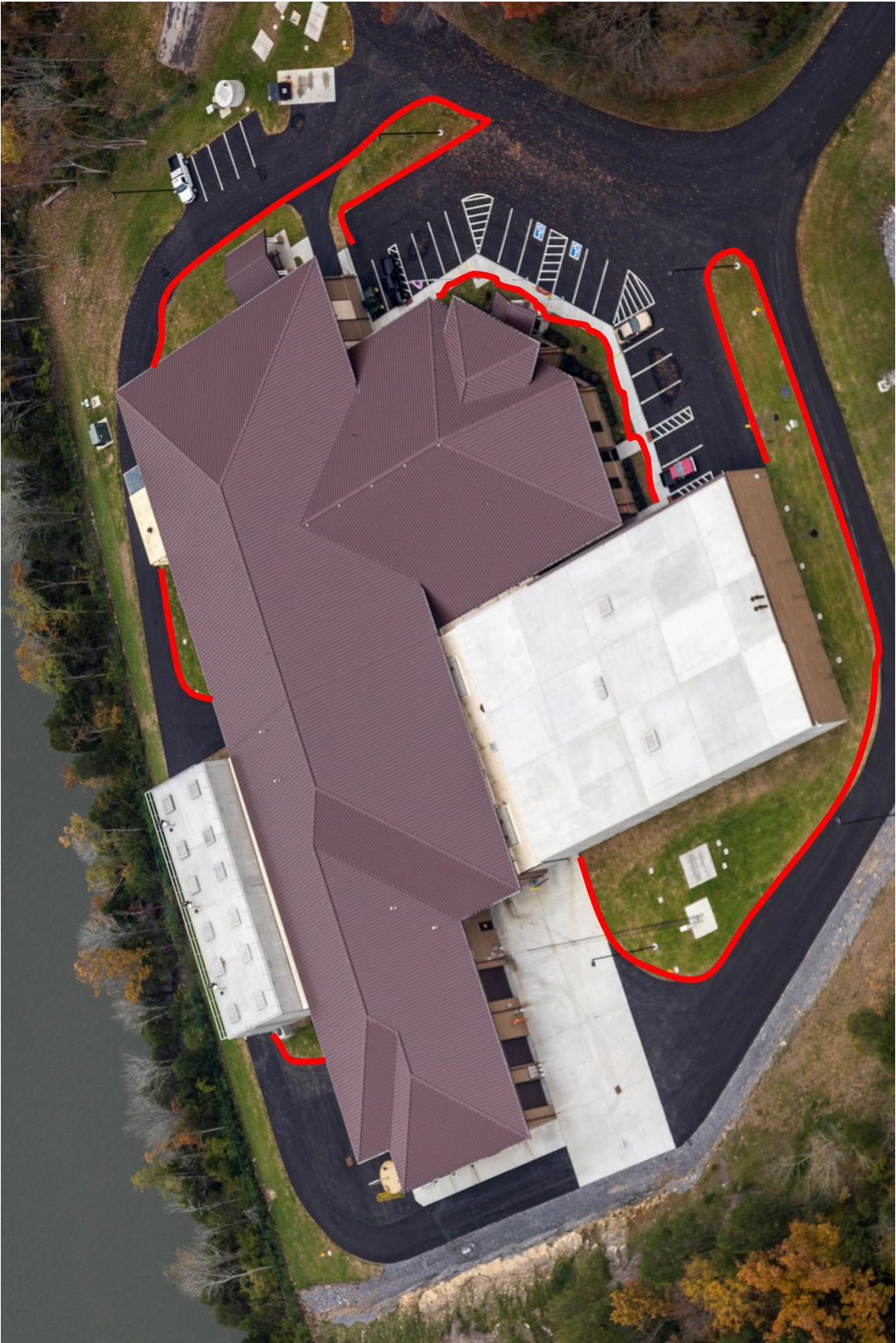
Water Treatment Plant, 131 Savo Bay
